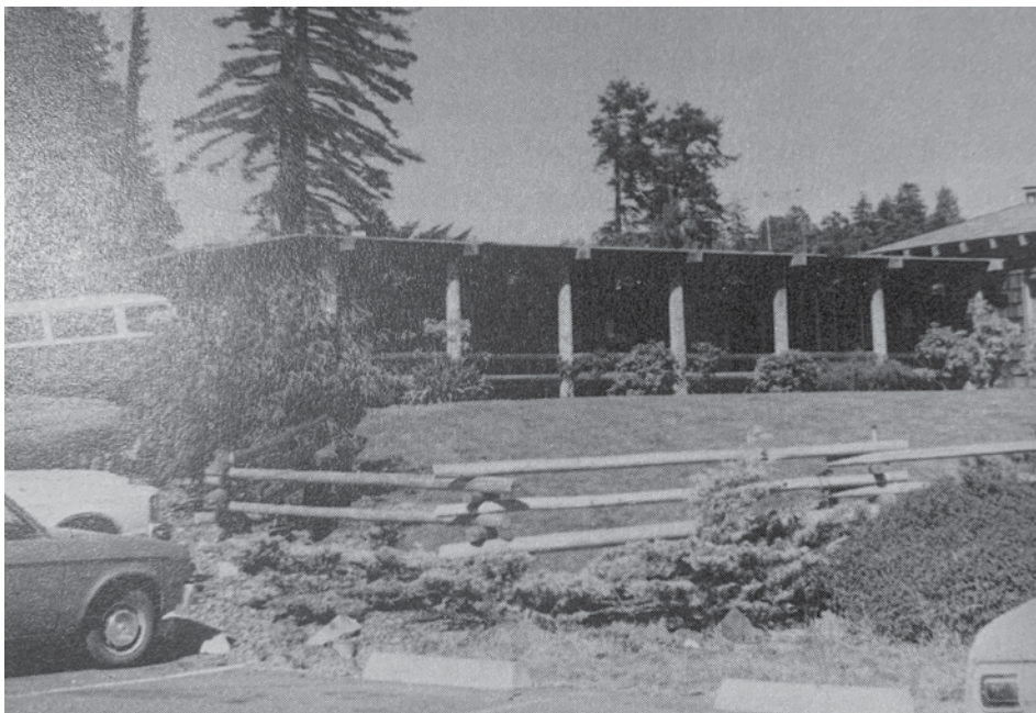
Tsurai Health Center in Trinidad - 1978
